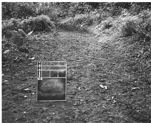
102 中山峠不陸整正工（施工後）図34-17
