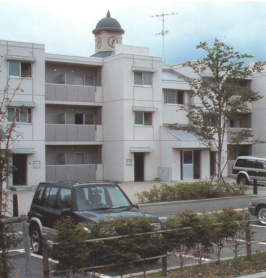
町営住宅 Town-operated housing
