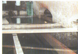
▲レンガ作りの貯水槽 Reservoir made of brick
